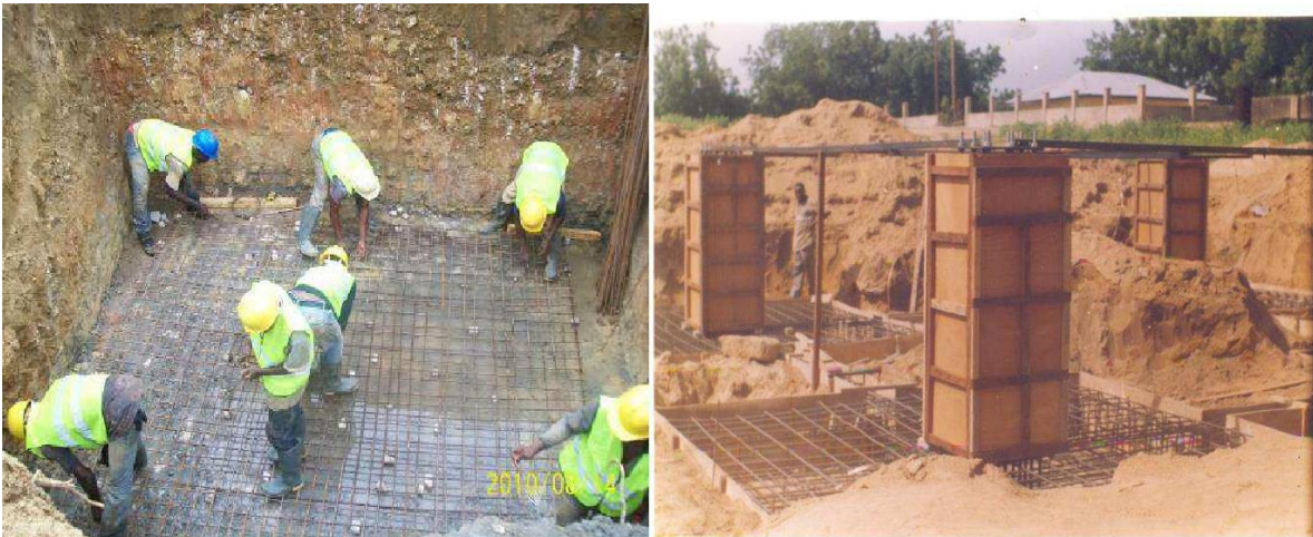
Typical GSM Tower Foundation under Construction
